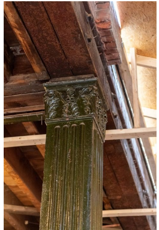
Original cast iron column to be part of the restored first floor commercial
