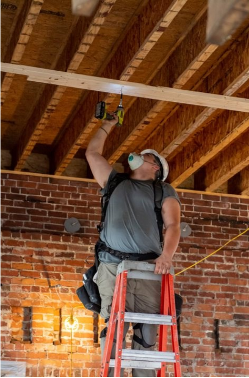
One of 50 construction workers on site from Bread Loaf Construction
