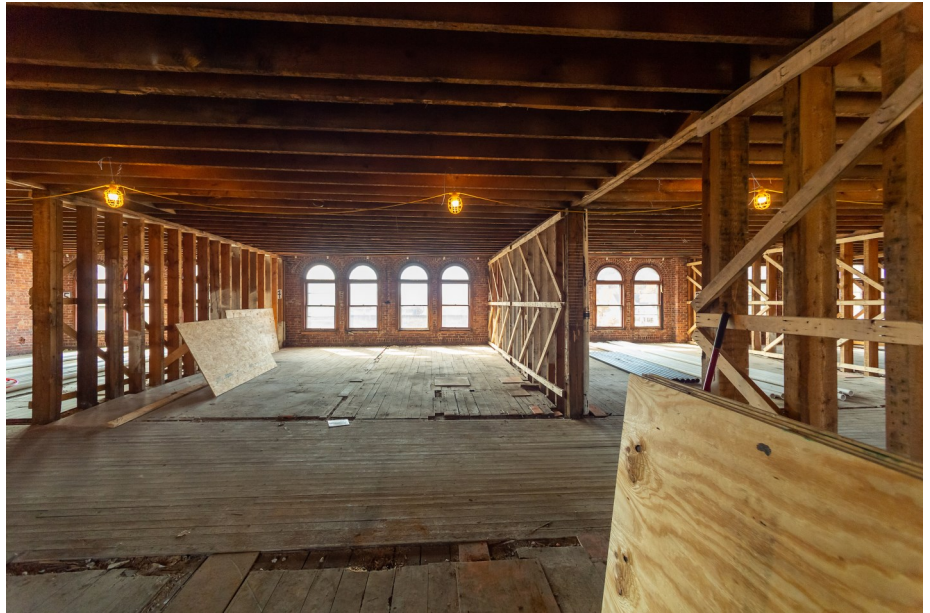
Starting interior framing
